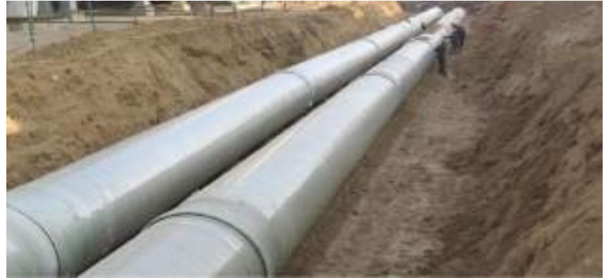
Circulating Water/Cooling Water Fiberglass Pipe Engineering Project of Shengli Power Plant, China Sinopec Model and Specification: DN1600, SN10000N/m 2
