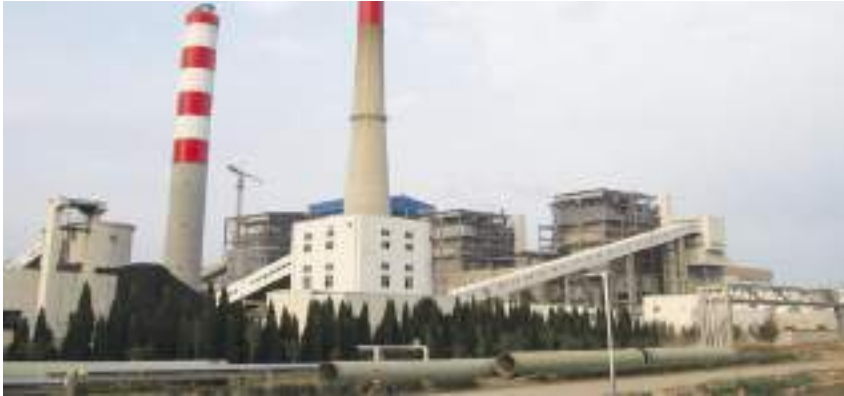
FRP Pipeline Project for Seawater Desulfuration in Shandong Rizhao Electric Power Plant Model and Specification: DN1400, SN10000N/m 2
