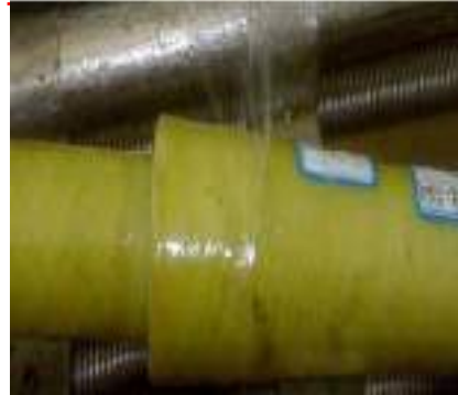
Joint leakage
