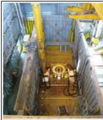
CONDUCTOR TENSIONING UNIT
